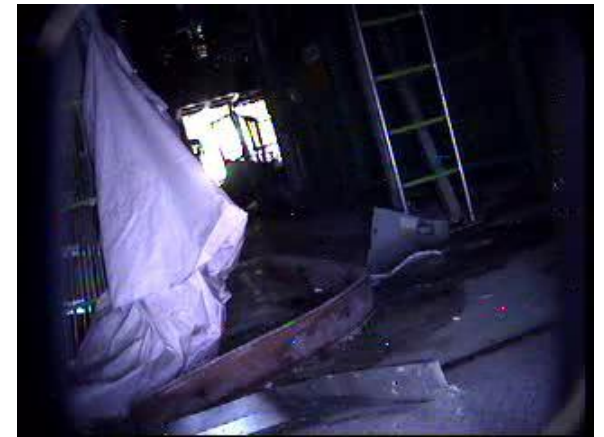
1 st floor of R/B Unit 3
