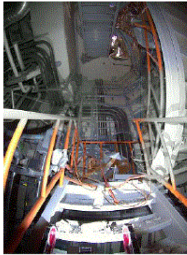
Staircase from 2nd floor to 3rd floor
