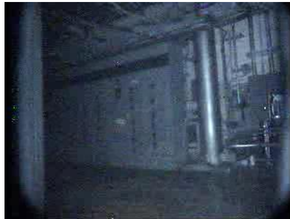
1 st floor of R/B Unit 2
