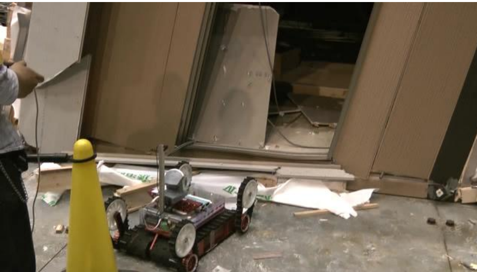
Entry into collapsed house
