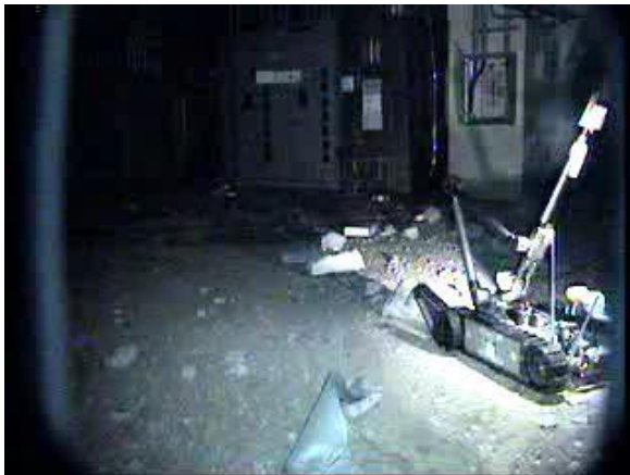
1 st floor of R/B Unit 1
