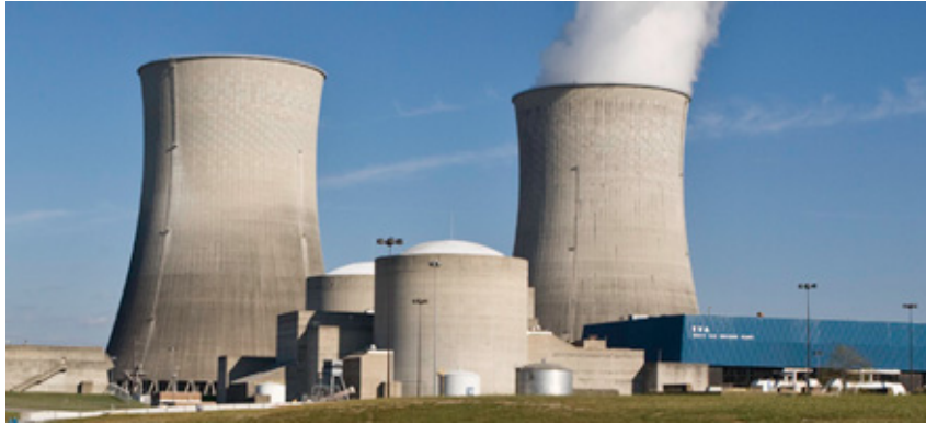
Figure C-1 Tennessee Valley Authority-Watts Bar Nuclear Power Plant
