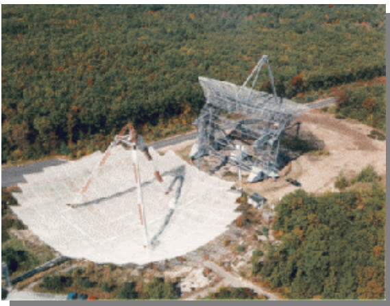
The two antennas of the Millstone Hill Radar at the Haystack Observatory in Massachusetts. Courtesy NSF's Division of Atmospheric Sciences.
