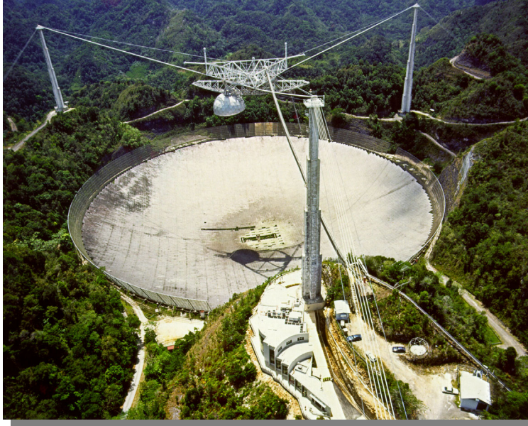
NSF's Arecibo Observatory, south of Arecibo, Puerto Rico. At 305 meters in diameter, Arecibo is by far the largest single-dish radio telescope in the world. It is used for radio astronomy, atmospheric/ionospheric research, and as a giant radar transmitter for mapping the structure of the Moon and planets. The telescope operates at various frequencies between 50 MHz and 10 GHz. Arecibo is operated by the National Astronomy and Ionosphere Center/Cornell University. (Photo courtesy NSF/NAIC/Cornell University).
