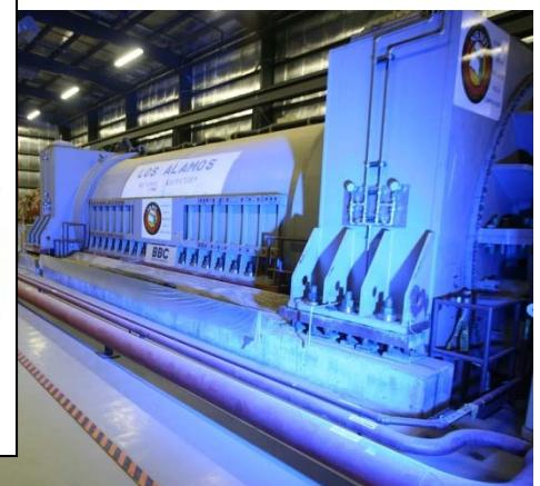
LANL's 1.43 GW generator can safely deliver a 600 MJ electrical pulse, a key capability giving the US a lead in high magnetic field generation capability
