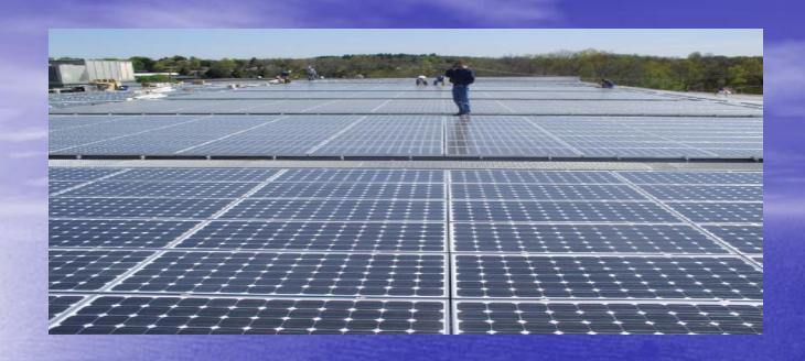
Solar Photovoltaic (Renewable Energy), The system on 31 Tannery using 1,276 Sharp 175W panels, producing 223 kWdc, using two Xantrex PV-100 inverters
