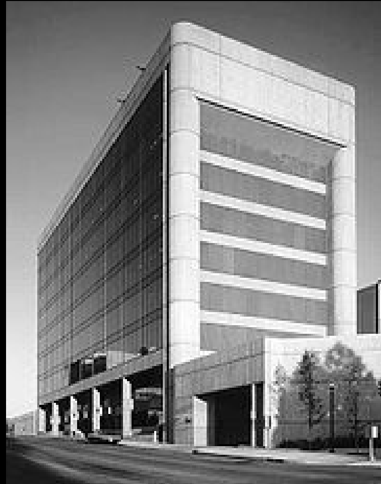
Alfred P. Murrah Federal Building
