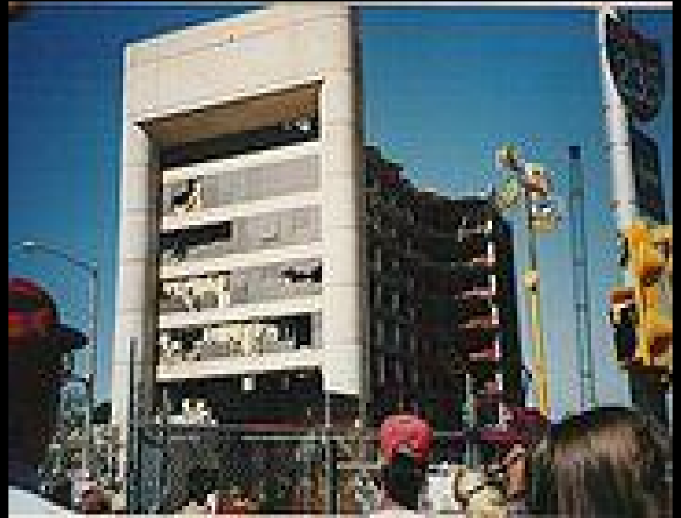
Murrah Building before demolition
