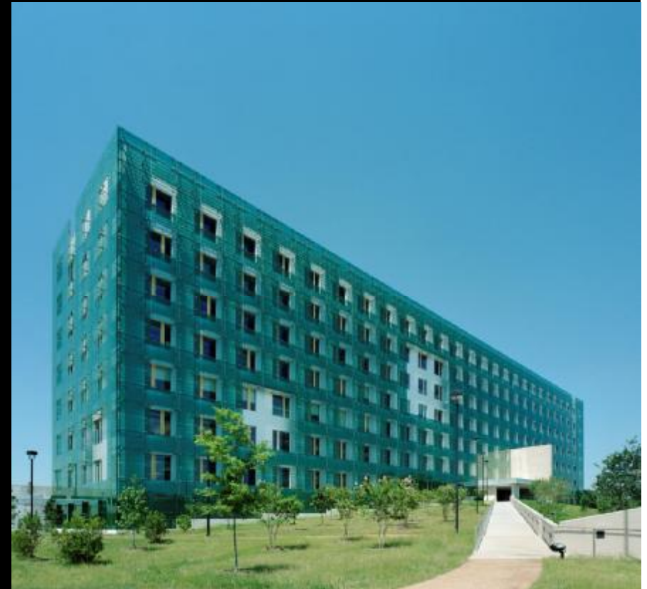
Concrete walls + second skin, punched windows
