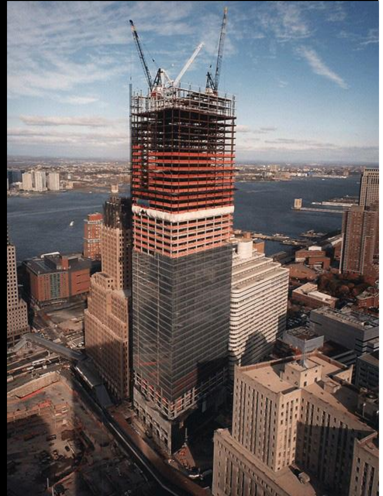
WTC under construction, 1960s
