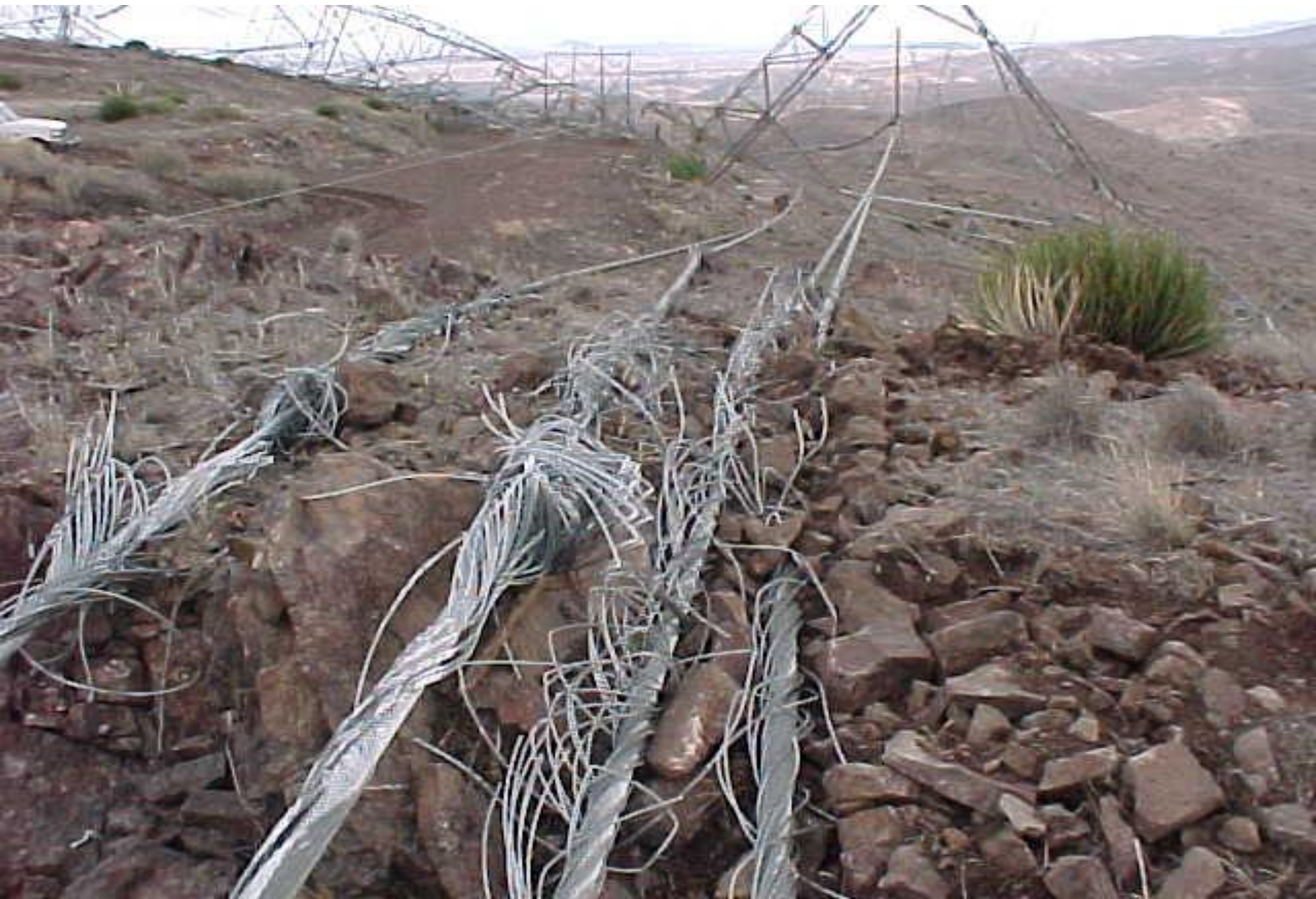
Midway – Vincent 500 kV line damage
