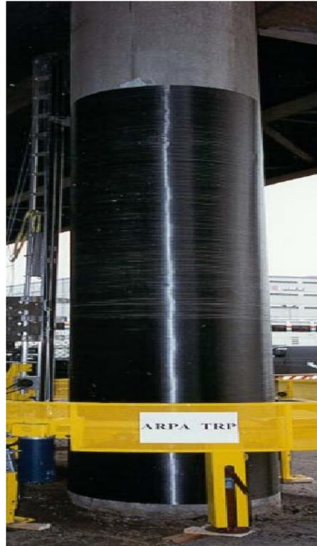
**Figure 10<sup>18</sup> Carbon fiber jacketing of a bridge column.**
