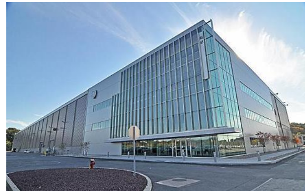
GE Battery Plant
