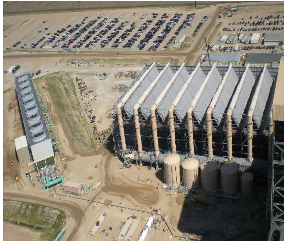
Comanche Power Plant
