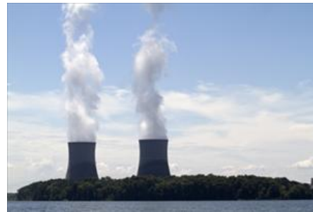
Cooling towers, TN
