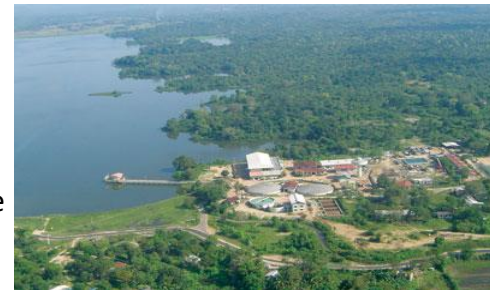
Cooling water intake
