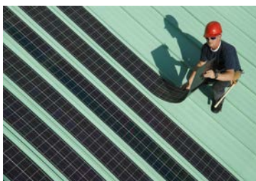
Figure 2. Installation of flexible solar panels for rooftop solar power generation 18
