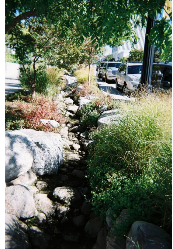
Figure 2: Portland's first Green Streets project at NE 35th and Siskiyou features curb cuts, bump outs and swales.
