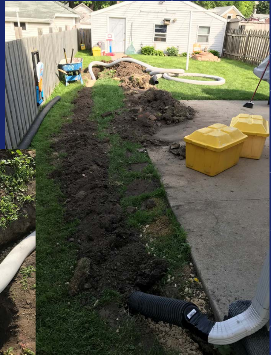
Sock covered drainage tile terminating in to drywell
