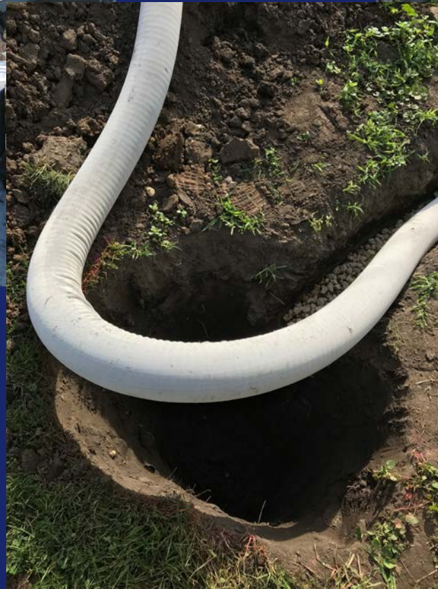
Sock covered drainage tile terminating in to drywell
