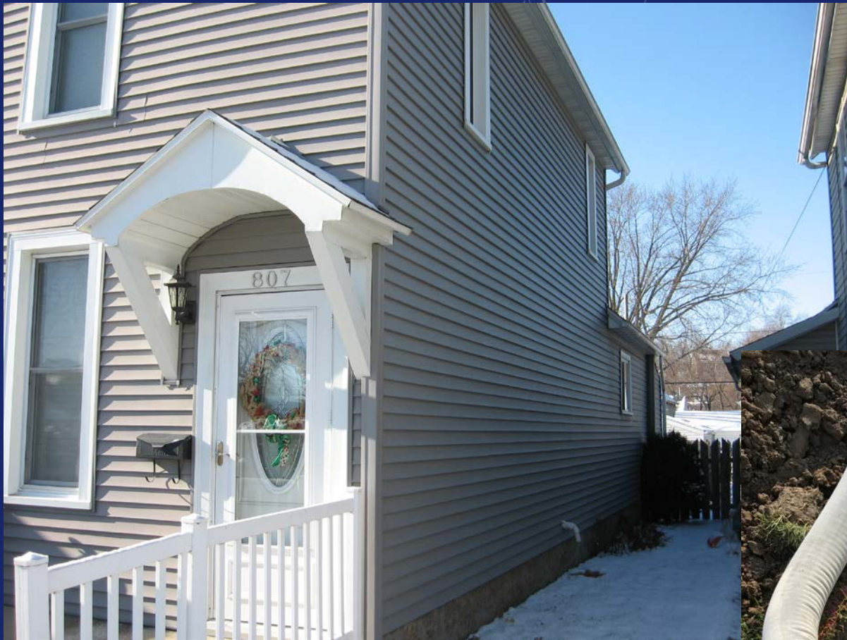
Existing gutter system draining to rear of home.
