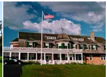
J. Erik Jonsson Conference Center 314 Quissett Ave Woods Hole, MA
