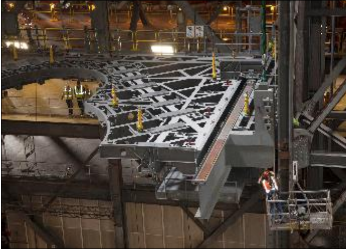
First Work Platform for Space Launch System Installed in Vehicle Assembly Building (VAB)
