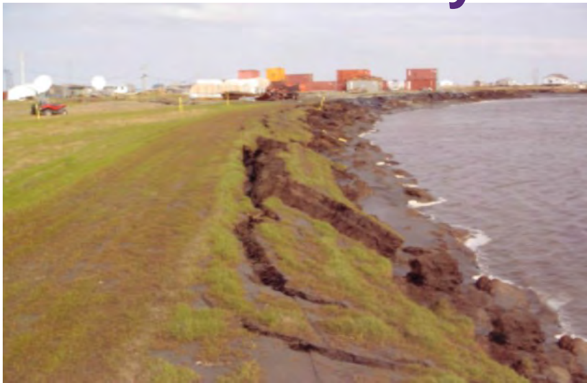
Kwigillingok: Erosion along barge landing site on Kuskokwim Bay in 2011. Yellow plastic poles are placed along the bank to measure rates of erosion.
