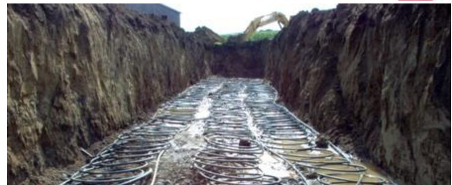
Geothermal Heat Pump System
