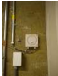
BAS Sensors (T/RH/Pressure)
