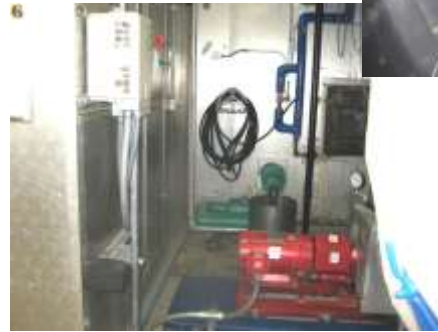
NEW PUMP VARIABLE FREQUENCY DRIVE
