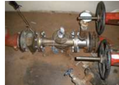
Water Meter & Sub-Meters
