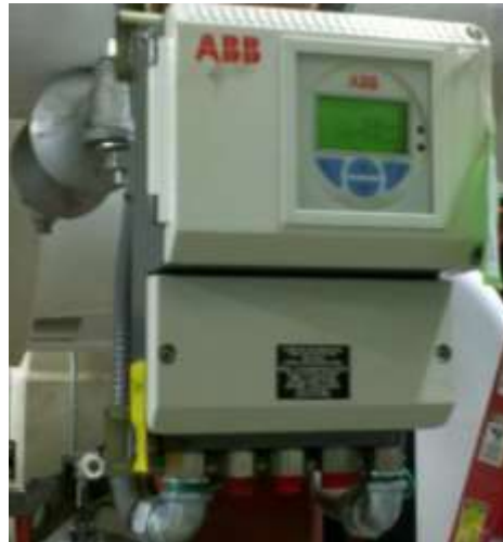
Chilled Water Sub-Meter
