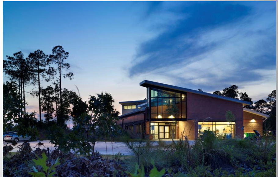
Community Emergency Service Station Fort Bragg, LEED Platinum
