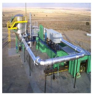
The Army's hazardous waste incinerators or APE 1236 M2 HWI, is used to demilitarize and/or dispose of ammunition items and bulk explosive wastes.
