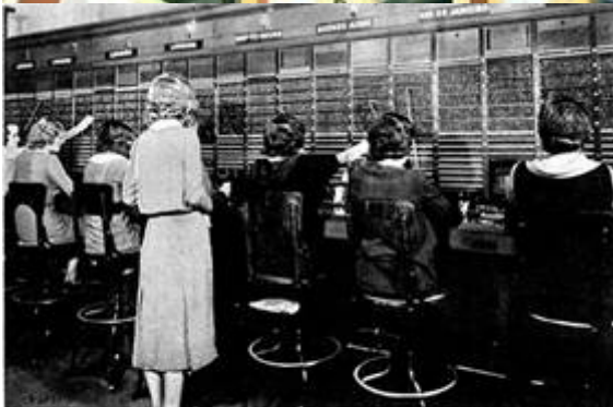
By courtesy of The American Telephone and Telegraph Co. A LONG-DISTANCE TELEPHONE EXCHANGE. Radio-telephone switchboard circa 1930. From the left the first four stations are to London, the next Ship to Shore, Buenos Aires, and Rio de Janeiro.
