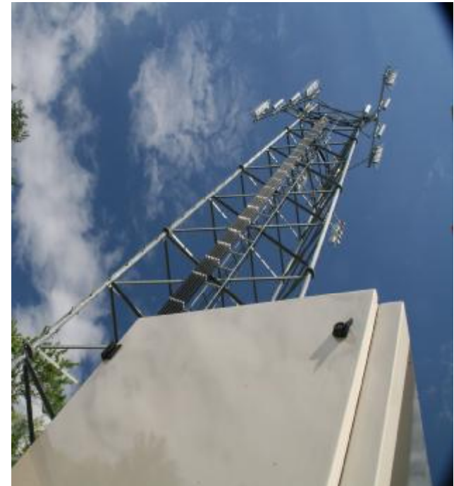
GenCore® 5T fuel cell system with cell tower
