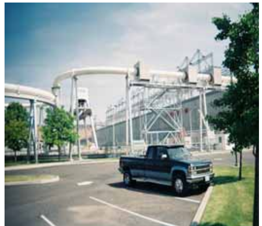
The Juvenile Bypass System at McNary Dam on the Columbia River
