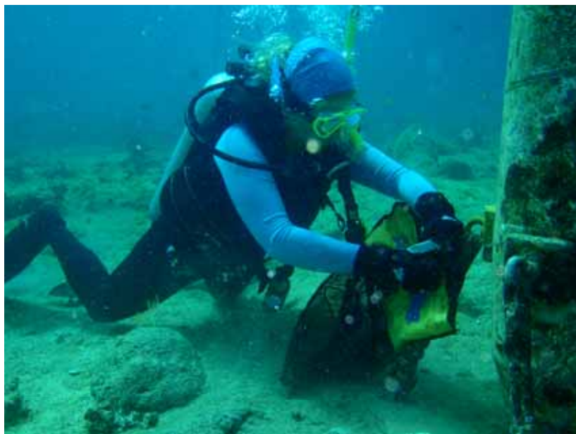
NOAA Corps officer of AOML works to clean away marine growth and other debris at the base of the St. Croix pylon.
