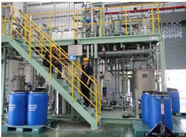
BDF Production Unit (1.0 ton-BDF/day)
