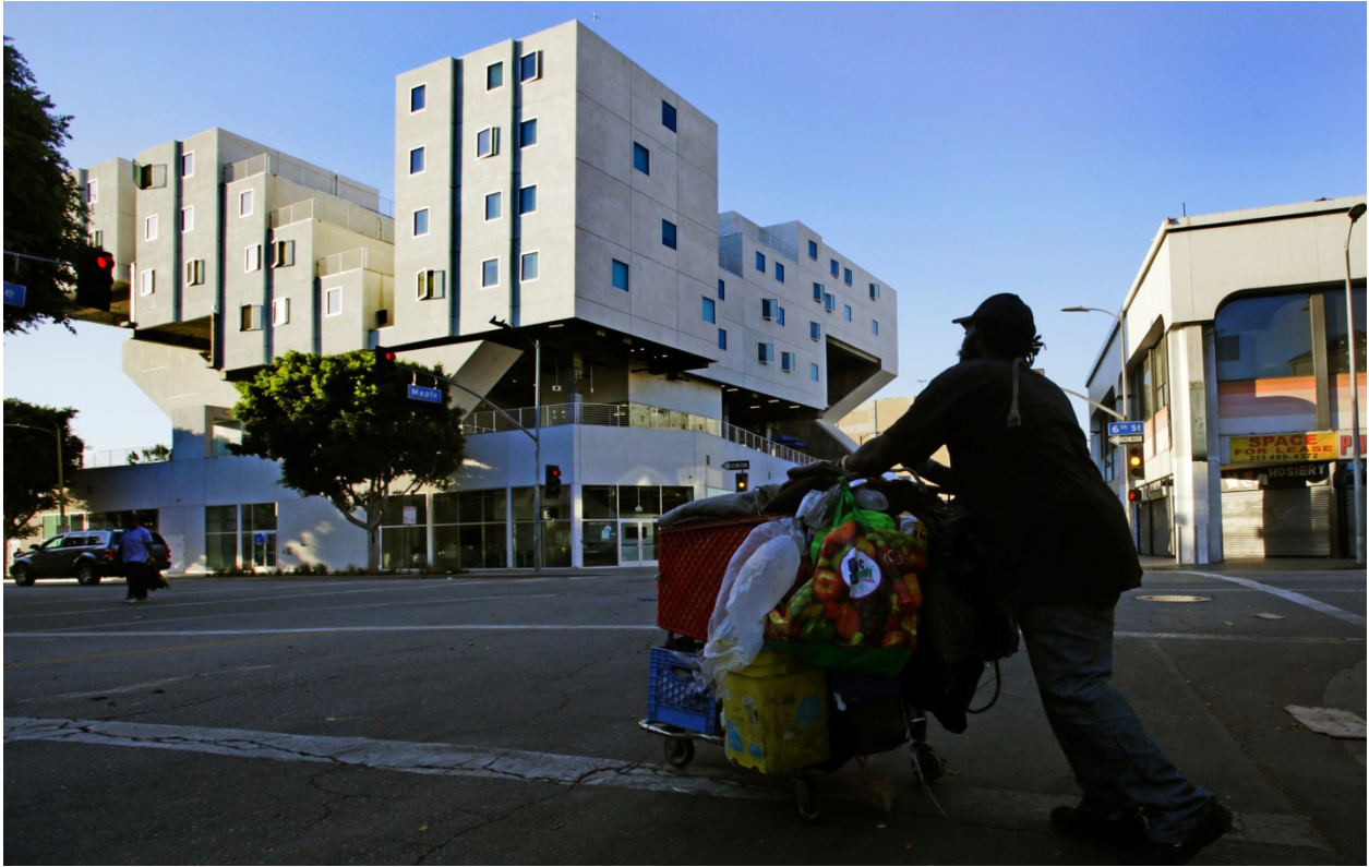
FIGURE 1 Star Apartments, Los Angeles, CA, built with funds from the Skid Row Housing Trust. SOURCE: Irfan Khan. Copyright © 2014. Los Angeles Times. Reprinted with Permission.
