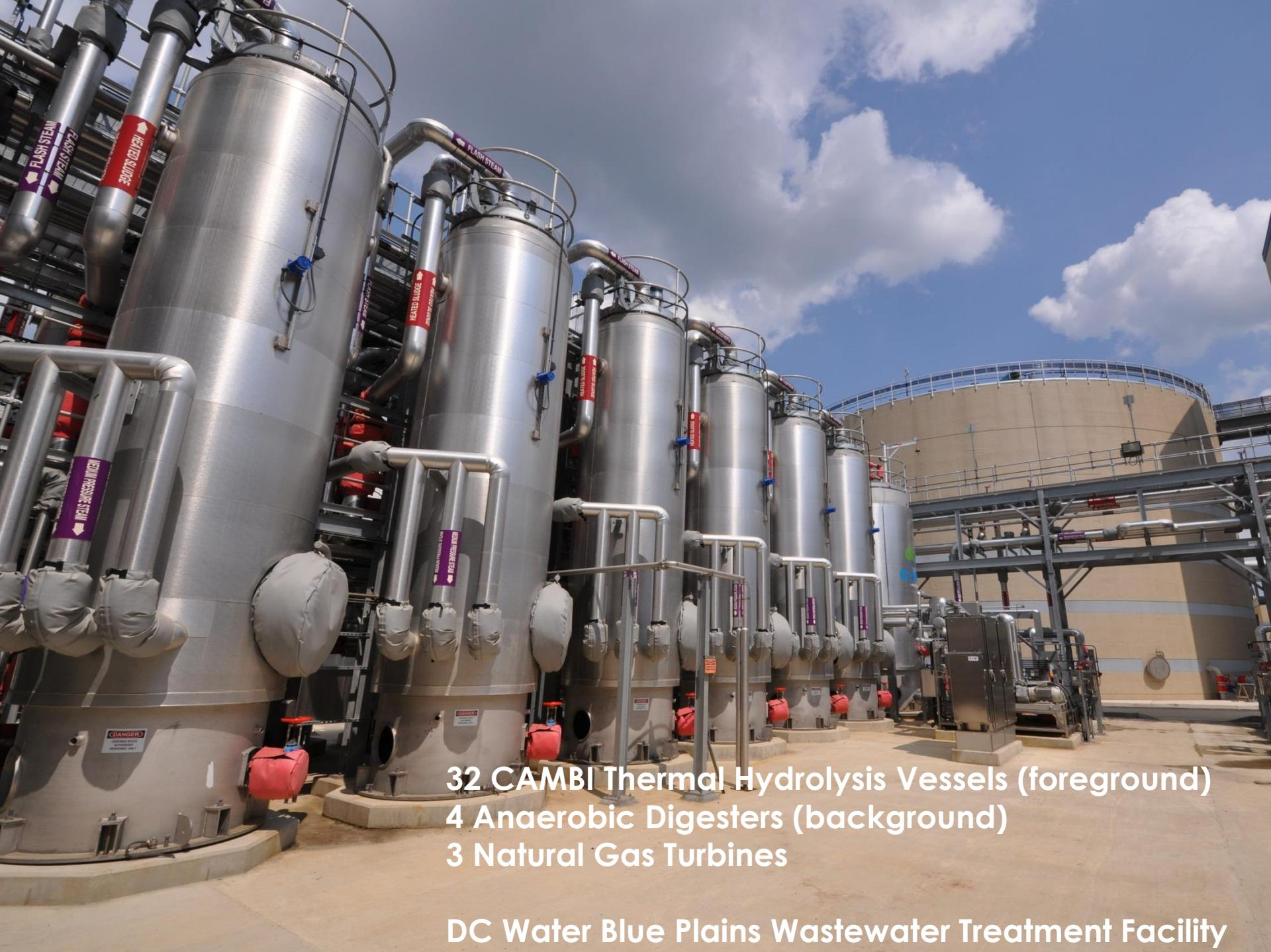
**32 CAMBI Thermal Hydrolysis Vessels (foreground)**
