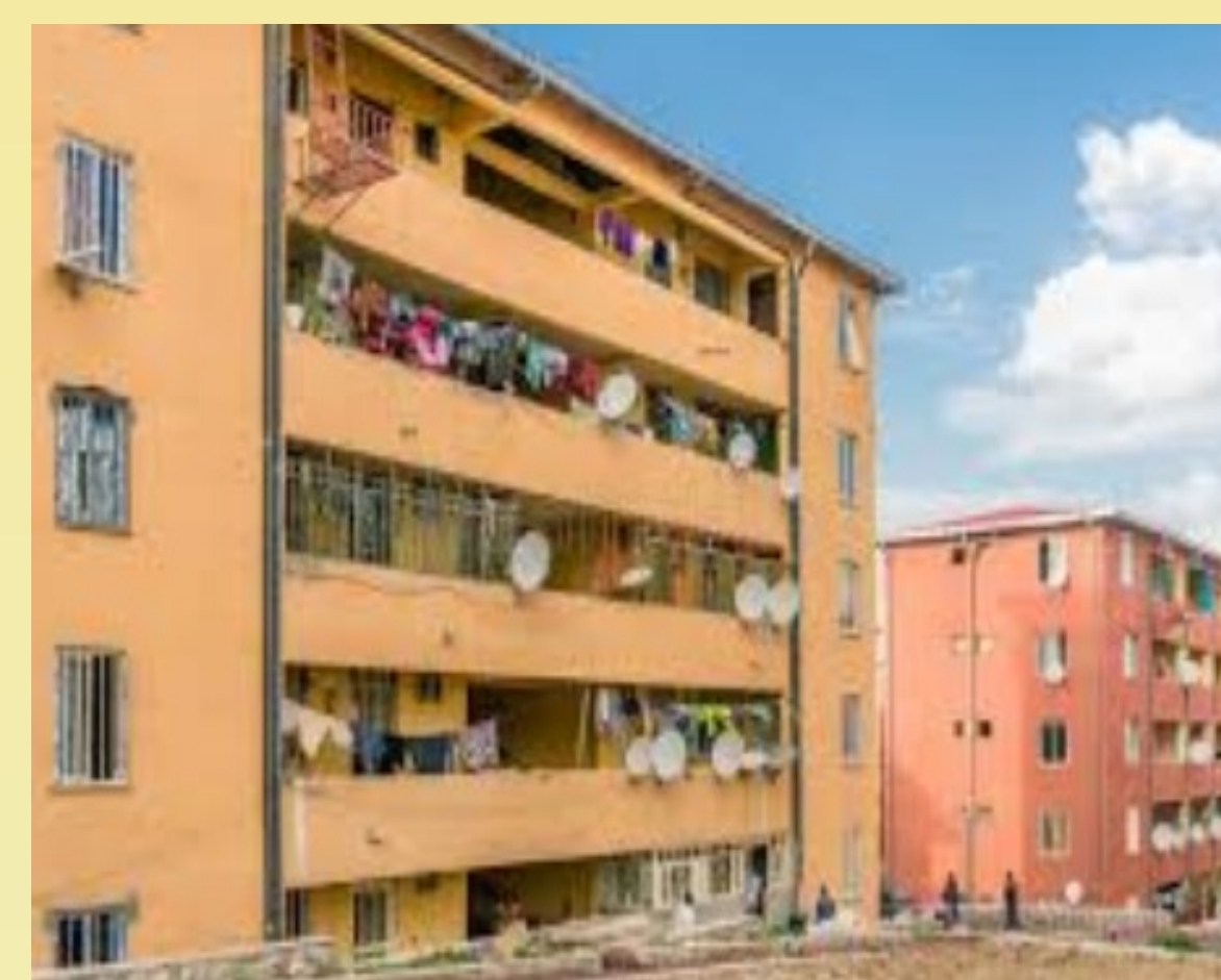
One of the condominium sites where MBR is applied for treatment of the wastewater
