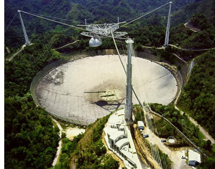
Arecibo (NAIC) 300 m antenna, 1 MW transmitter, 13 cm wavelength (S band)
